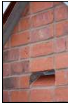
Figure 2: Habitat Bat Box faced with red brick, incorporated within wall at gable end.
