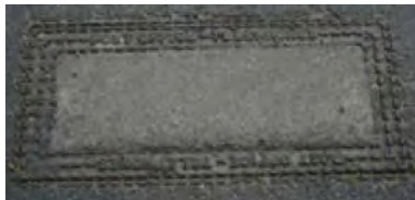
Old style cast iron and concrete 38x80cm
