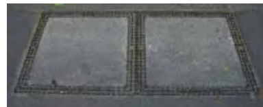
JF6 old cast and concrete type 70x140cm
